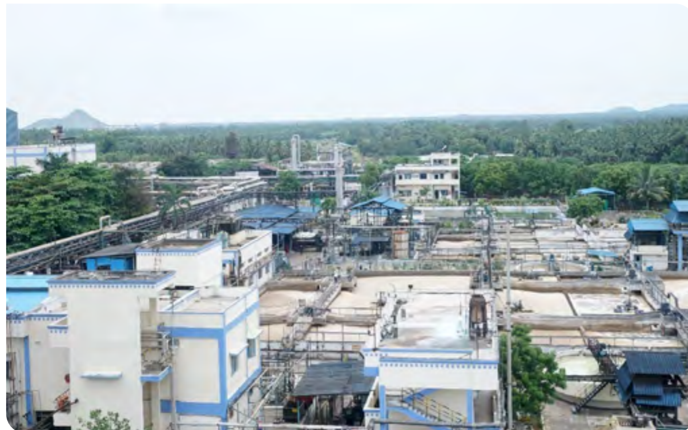
Effluent Treatment Plant
