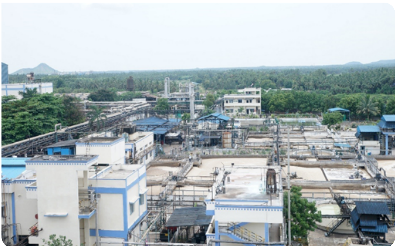
Effluent Treatment Plant
